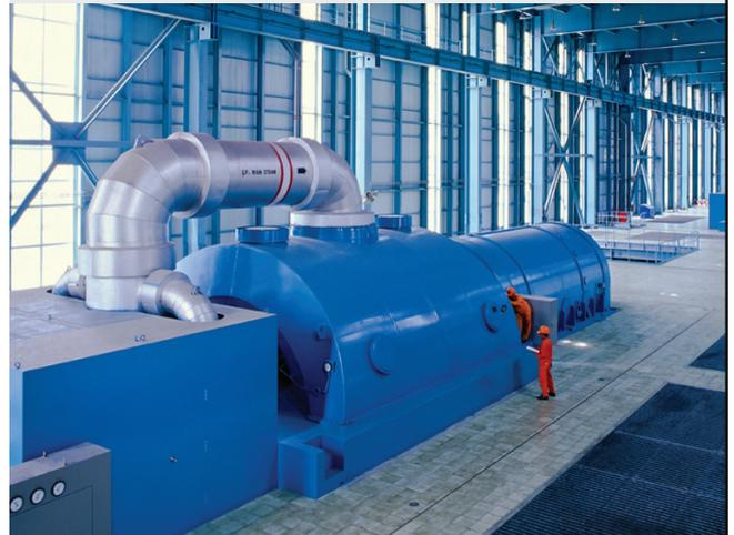
Hydrogen cooled power generators operate more efficiently and are often more cost effective than air cooled counterparts.
