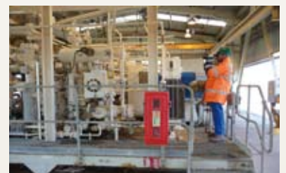
Using GasFindIR HSX to check for natural gasleaks
