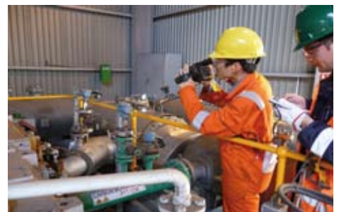
In both pictures CO leaks were found with the GasFindIR CO
