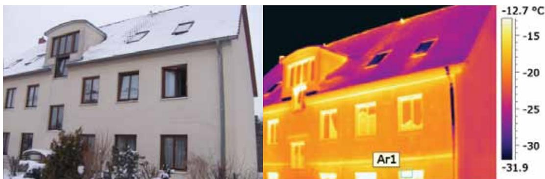
*In this example it is clear that the rightmost skylight is leaking warmth at the frame and there are several locations where the roof insulation isn't very effective.*
