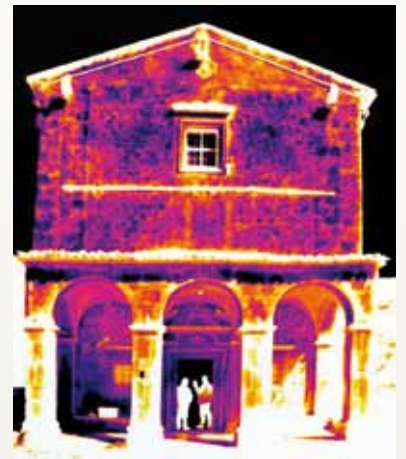
Picture of the S. Stefano di Sessanio (AQ) church, before and after the earthquake
