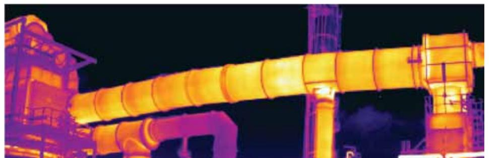
Hot spots on these ducts indicate faulty insulation.
