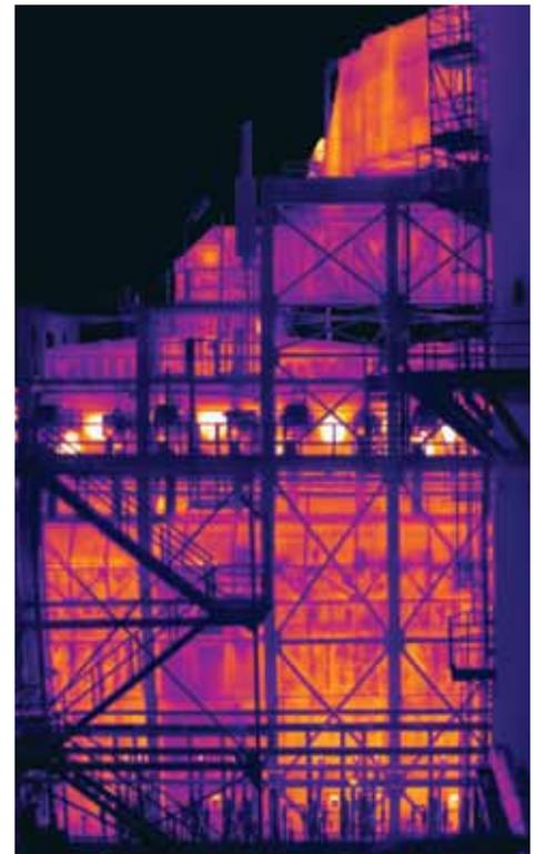
A cabin furnace as seen from a distance of about 80 meters using the FLIR P640 thermal imaging camera.
