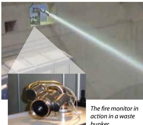
*The fire monitor in action in a waste bunker.*
