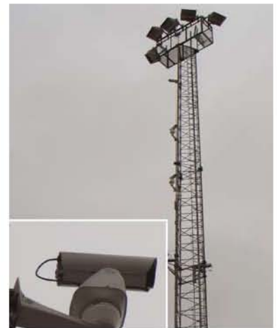
Typical airport thermal camera installation
