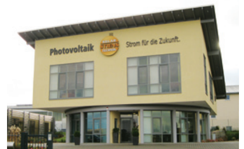
Every 10 minutes the upper story of the main office building of Solartechnik Stiens in Kaufungen moves almost imperceptibly, directing the solar panels on the roof toward the sun.
