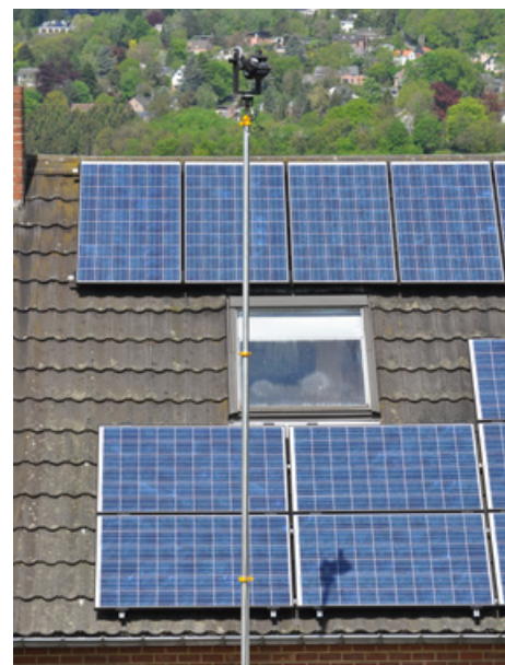
The aluminum pole is approximately 12 meters high, allowing it to inspect the roofs of most residential homes.
