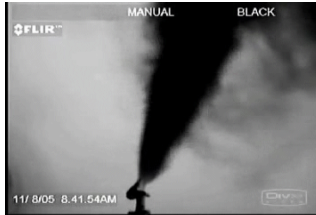
Figure 8, Failed rupture disk. Quantified annual leak rate of $1M.
