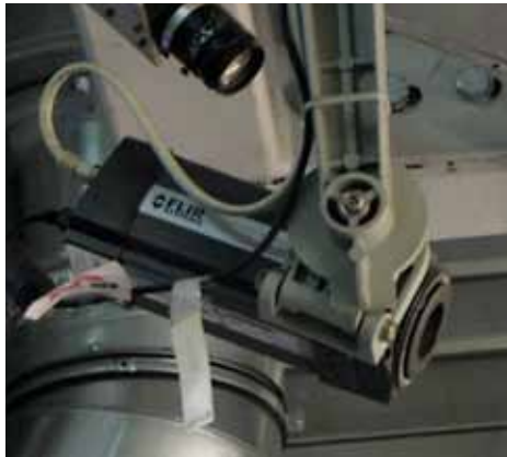
This FLIR A320 thermal imaging camera is used to check the front window heating system for defective heating elements.
